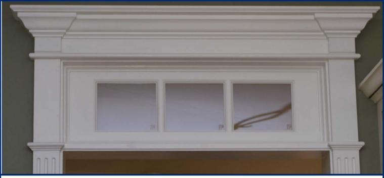
Sizing Formula: inside to inside of jambs + 1/2"(2-reveals)+ 2x pilaster width
